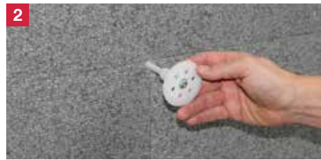
Insert the anchor with pre-mounted screw into the drill hole until the washer rests slightly on the surface
