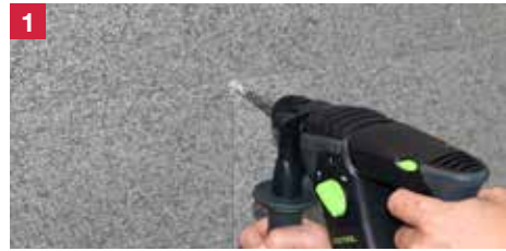
Quick drilling thanks to reduced drill depth
